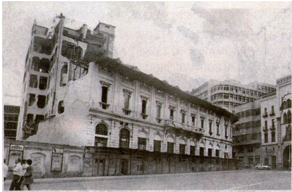
Figure 2: Former Hotel Alférez Real Demolition Source: https://repository.icesi.edu.co/items/5f9b8cea-3679-7785-e053-2cc003c84dc5
