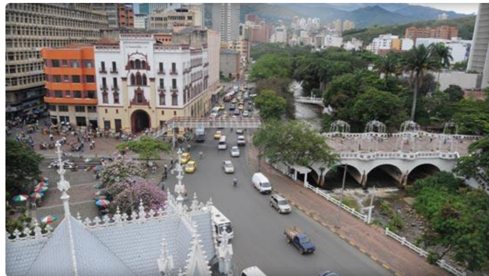
Figure 1-2: Avenida Colombia before Intervention
